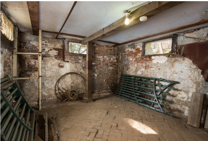
The basement of the Workman House.
