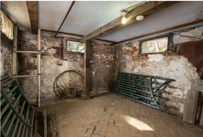
The basement of the Workman House.
